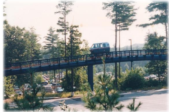
Full-scale track structure for testing and display
