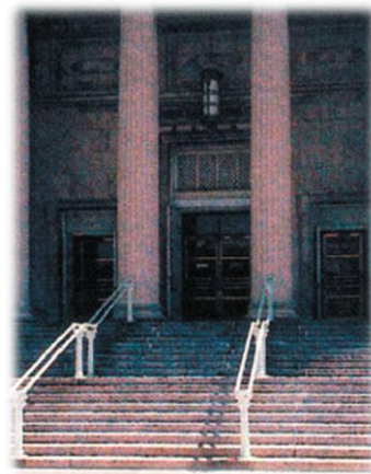
Nearest Entrance to Metra Station Closed, No Signs
